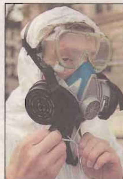
Warren Westura/Special to the Herald News Scott Krellick and John Klinkose, top, open the tenting around the statue of Garret Hobart outside Paterson City Hall. They will clean the statue's surface by "walnutblasting" it, using ground walnut shells, above left, instead of sand because the shells are less abrasive to bronze. Klunkose, right, puts on a protective suit and mask.
